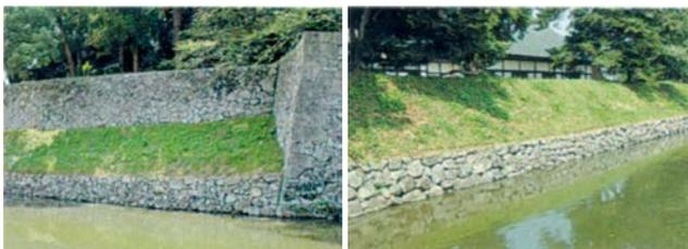
**Figure 9:** Inner Moat Stonework. Around the lower part of the earthen embankment known as Hachimaki Ishigaki (“Hachimaki” means headband) and Koshimaki Ishigaki (“Koshimaki” means waistband type underwearing of women). This type of stonework is rarely seen in the Kansai region, southwest Japan.
