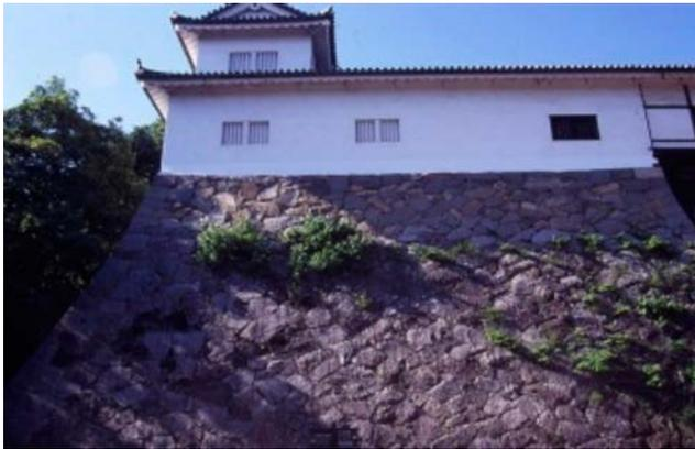
**Figure 7:** Stonework of Hikone Castle. Two-storied turret at the gates, which has been repaired many times, especially in 1854. The stone wall of right hand side was made in the original Gobozumi style of stone work. The left side was made by the later Otoshizumi style, because it was destroyed by the earthquake and re-built.
